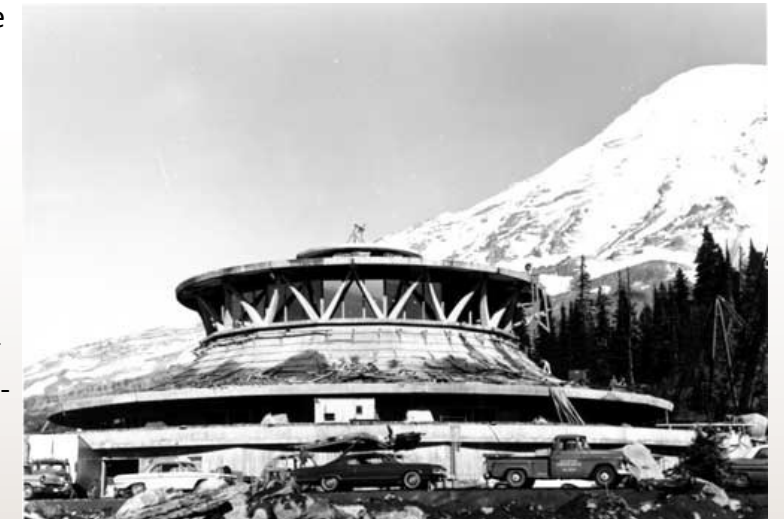
Old Jackson Visitor Center under Construction
